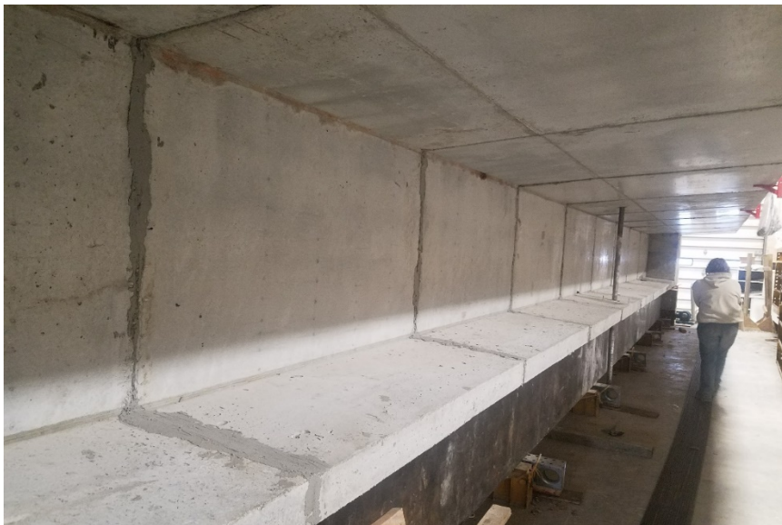
Figure 3.9 – Joint Interfaces after Curing (Sritharan et. al., 2018)
