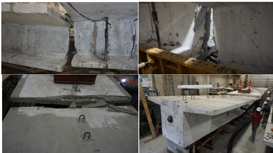
Figure 3.30 - Girder BON2 after Failure (Sritharan et. al., 2018)
