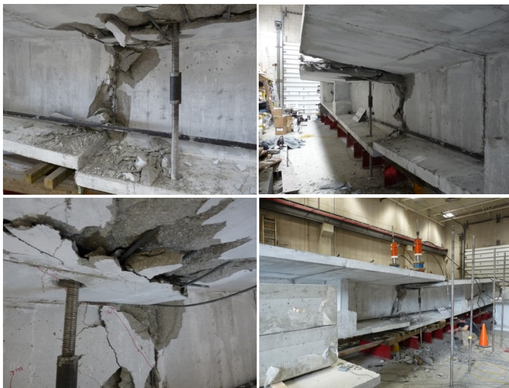
Figure 3.26 – Failure Mode of UNB3 (Sritharan et. al., 2018)
